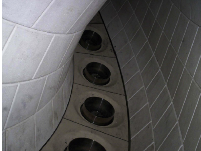
Figure 1.4: A DLN annular combustor in a Siemens V94.3 Gas Turbine.
