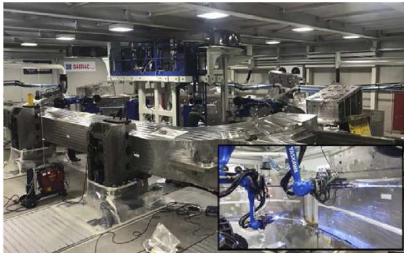
Figure 18: Coil Cases welding [37].
