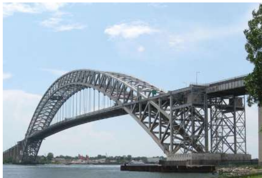
* The Bayonne Bridge (FR)
